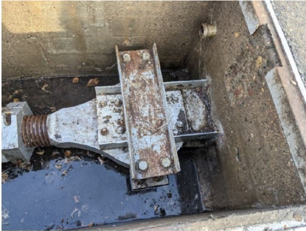
Figure 1. Aerial of MG Anchorage pit
