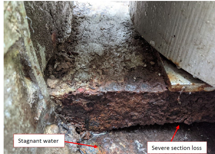
Figure 4. Section loss in bottom plate at LD 3
